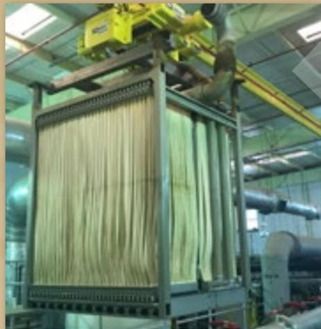
A cassette from our Membrane Treatment Plant. Each cassette has thousands of hollow fibers that filter dirt, debris, and micro-organisms out of the water.
